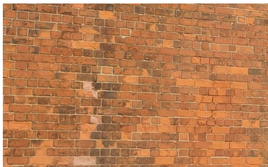
Photo 27: Brick wall in English Bond having alternating courses of headers and stretchers
